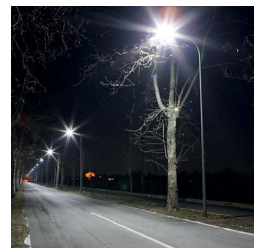
BEFORE - 100 W HP SODIUM LAMP AFTER - 66 W LEDs
